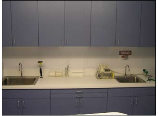
Hands-free sinks for instruments help prevent cross contamination.
